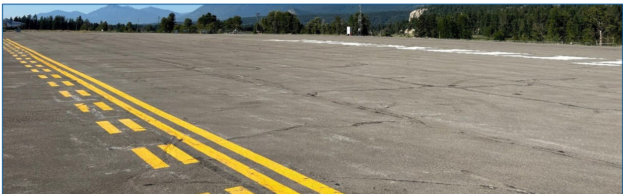
Taxiway A – Apron I intersection
