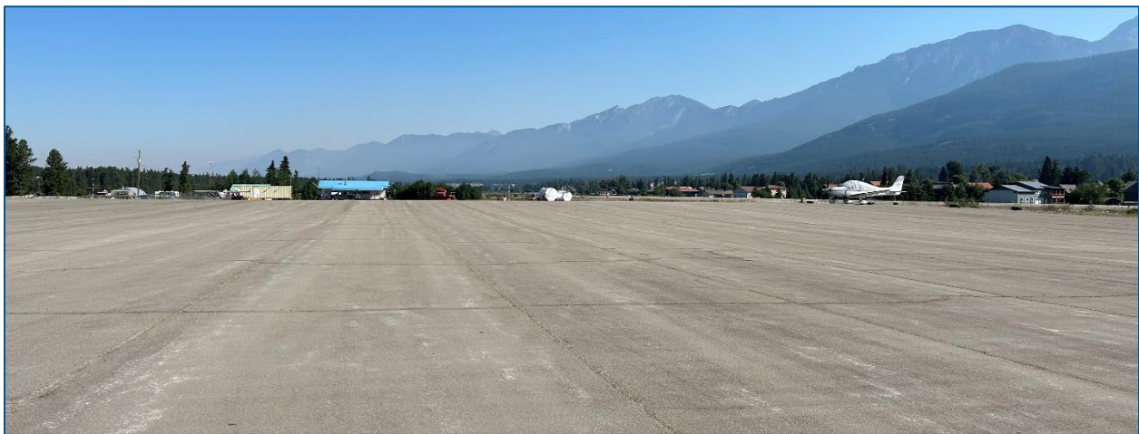
Apron I overview, facing north
