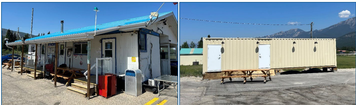
Office building (left) and washroom facility during installation (right)
